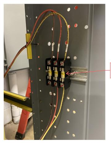
15A Fuses - DIN rail mounted for Power Quality Meter Circuit
